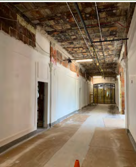
Old Cook County Hospital Administration Building, Chicago IL-HTC Project
