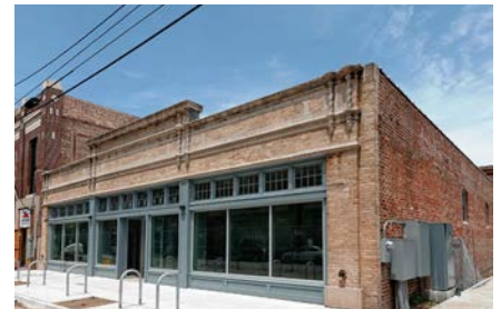
Photo credits: FH Myers Construction
