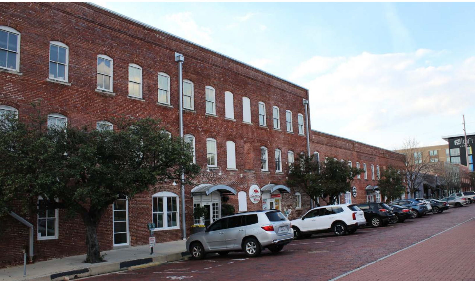
West Gervais Historic Commercial District
