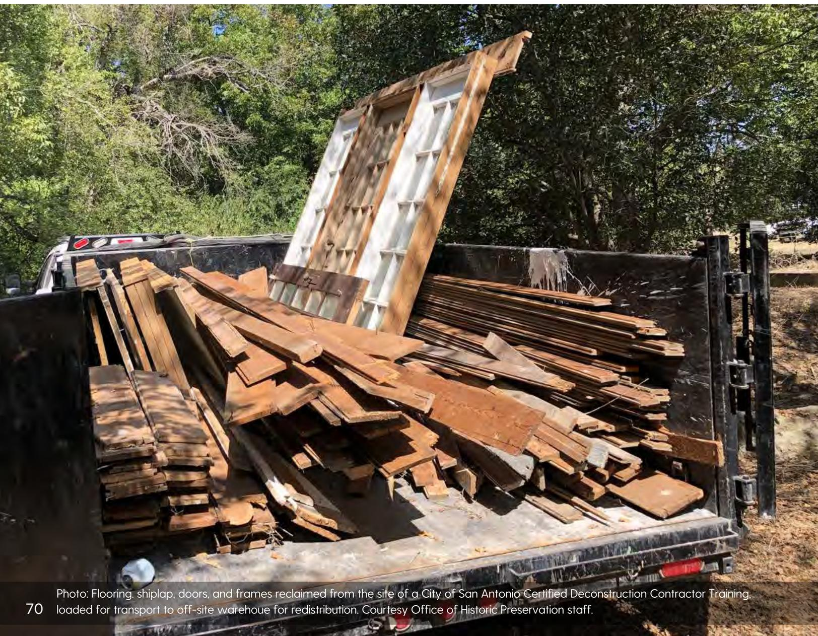
Photo: Flooring, shiplap, doors, and frames reclaimed from the site of a City of San Antonio Certified Deconstruction Contractor Training, loaded for transport to off-site warehouse for redistribution. Courtesy Office of Historic Preservation staff.
