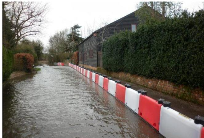
**Figure 4.15** Quick Deployable Flood Barrier (Fluvial Innovations 2020)
