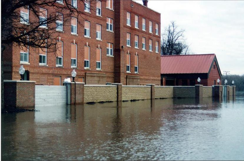
**Figure 4.8** Masonry Floodwall with Engineered Temporary Flood Gates (FEMA 2013)
